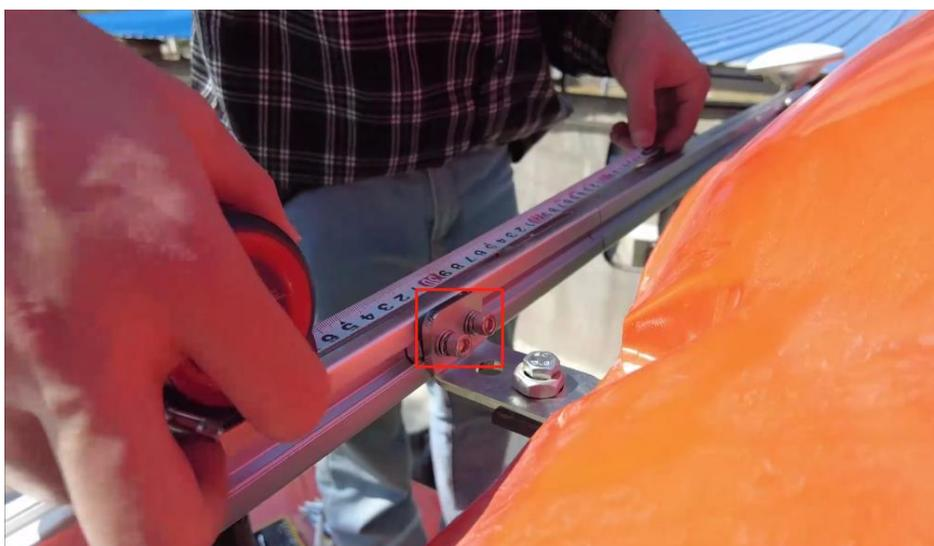
Figure 2.1.18 Crossbar fixing
