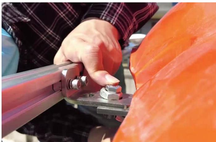
Figure 2.1.17 Sliding mounting plates fixing
