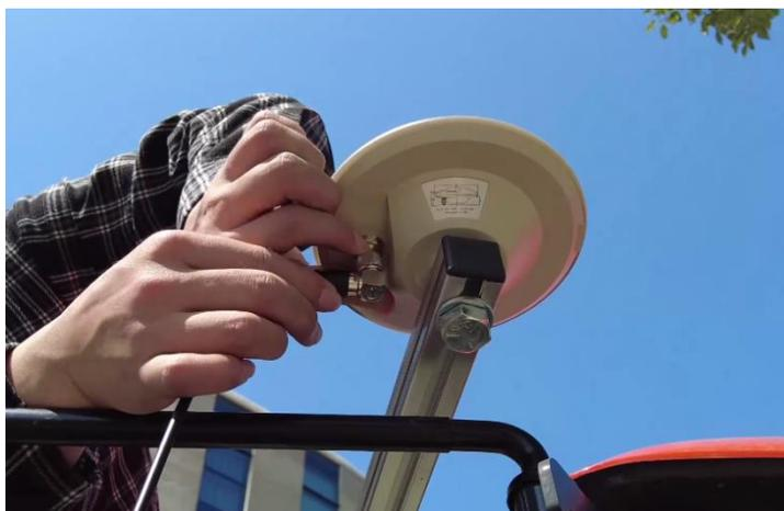
Figure 2.1.19 Antenna cables connection
